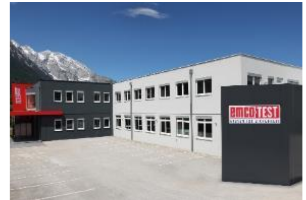
Production facility in Kuchl
